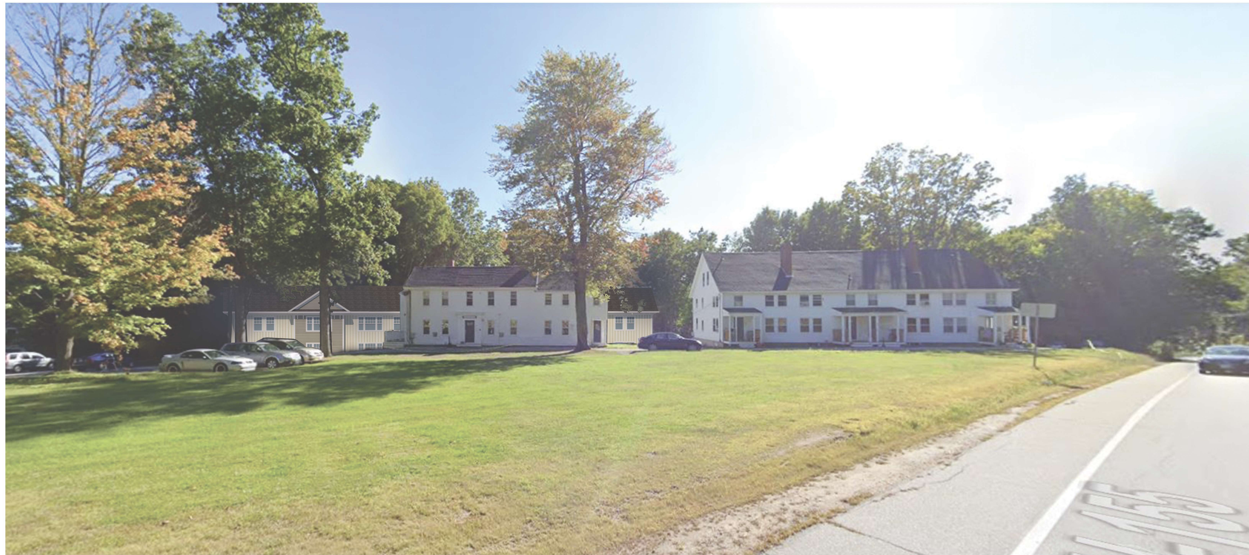
VIEW FROM LEE ROAD AT FRONT OF EXISTING BUILDINGS
